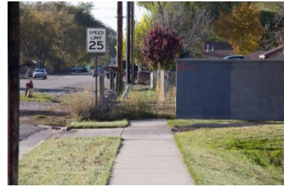
Incomplete Sidewalk, West Valley City
